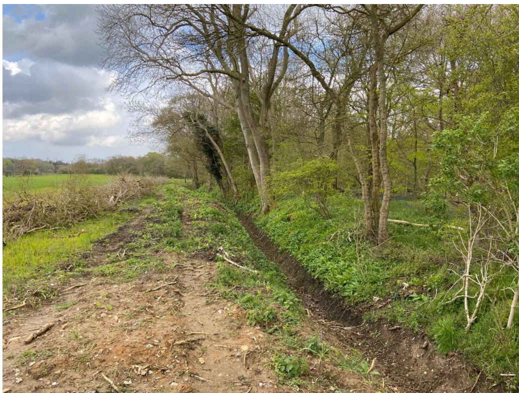
Photograph 7. Recently re-excavated ditch at western margin of Foxburrow Wood
